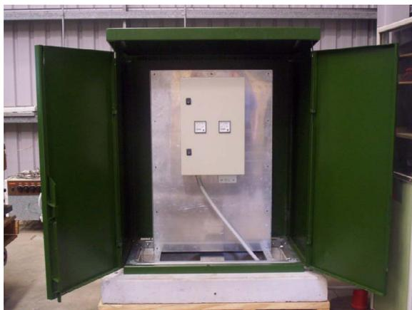
Fig16. SWER Voltage Controlled Reactor System
