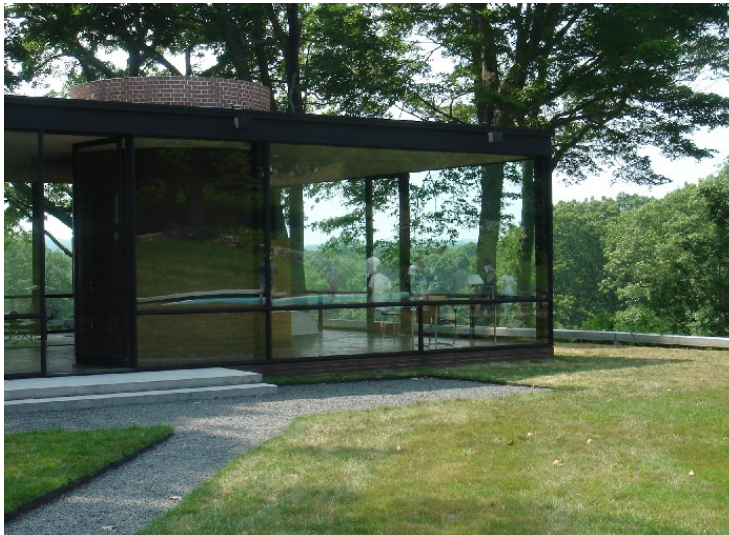
Figure 5: Philip Johnson's 1949 Glass House in New Canaan, Connecticut. The house is raised above the landscape on a brick podium; its interior space clearly demarcated by glass, steel, and concrete steps, from the meticulously manicured lawn outside. Photo copyright: D.J. Huppertz
