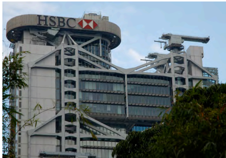
Figure 46. Window cleaning mechanisms on the HSBC building.
