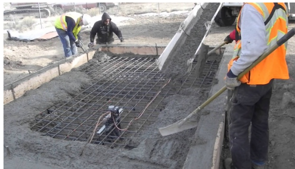
Figure 1. 1: Concrete poured over steel reinforcement (American Concrete Institute)
