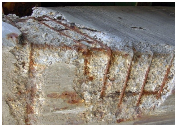
Figure 1. 3: Typical view of corrosion of steel reinforcement (spalling) in concrete (ACI)
