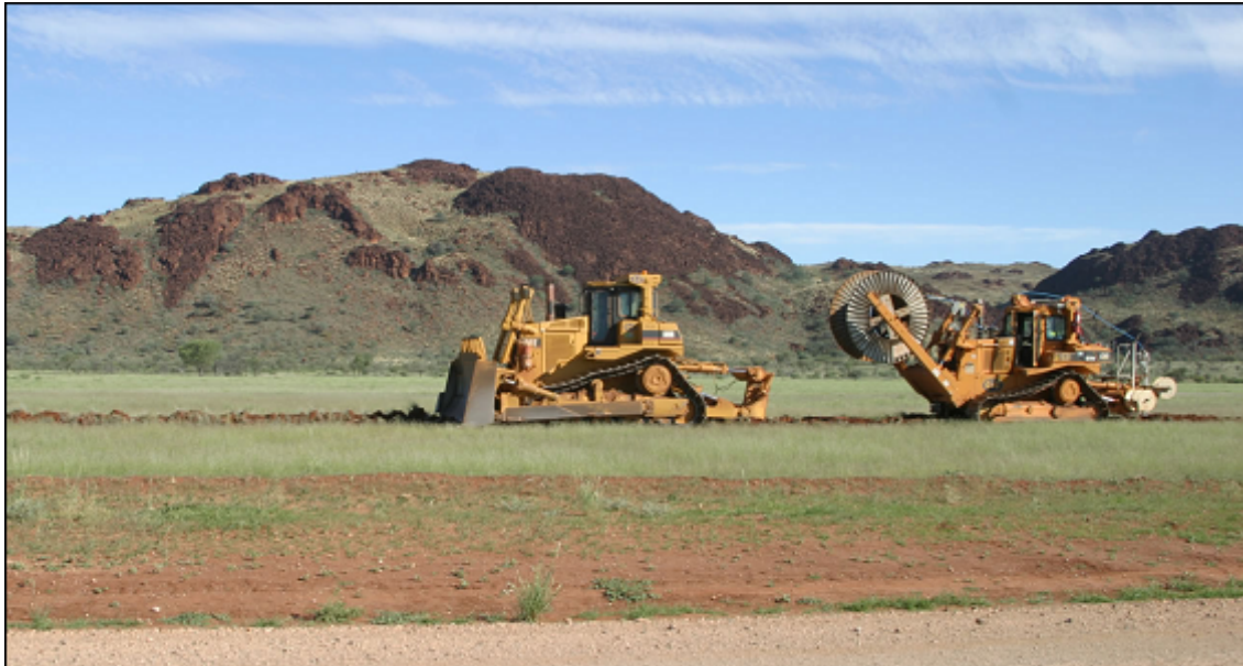
Figure 4 - The fibre optic cable being laid near Blackstone community. (Photo: Daniel Featherstone/ Ngaanyatjarra Media)
