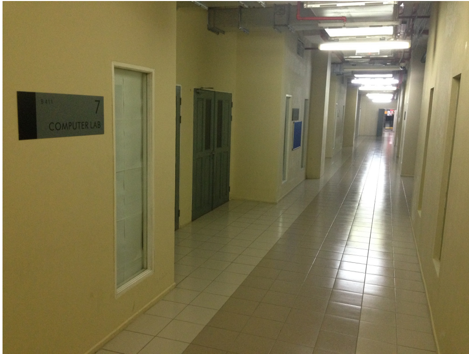
Fig. 3.2 Long corridor of site no.1.
