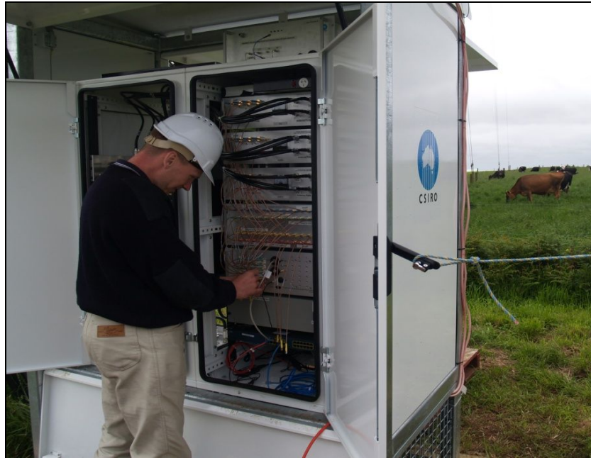
Figure 4 - Photograph of access point units.
