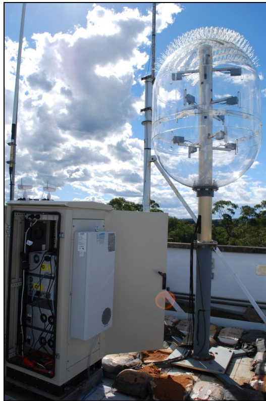
Figure 11 - Access point antenna array (right) and outdoor enclosure (left) installed on the rooftop of CSIRO Radio Physics Laboratory building in Marsfield.
