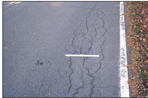
(b) Medium Severity Cracking
