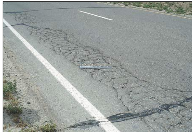
(c) High severity cracking
