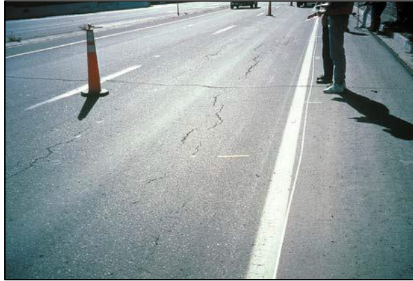
(a) Low severity cracking
