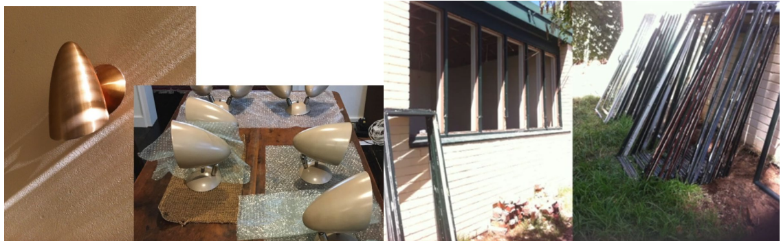
Fig.6.16 Atomic lights, that were upcycled and re-fitted-to the left, and the original steel windows which were reconditioned and reused-to the right
