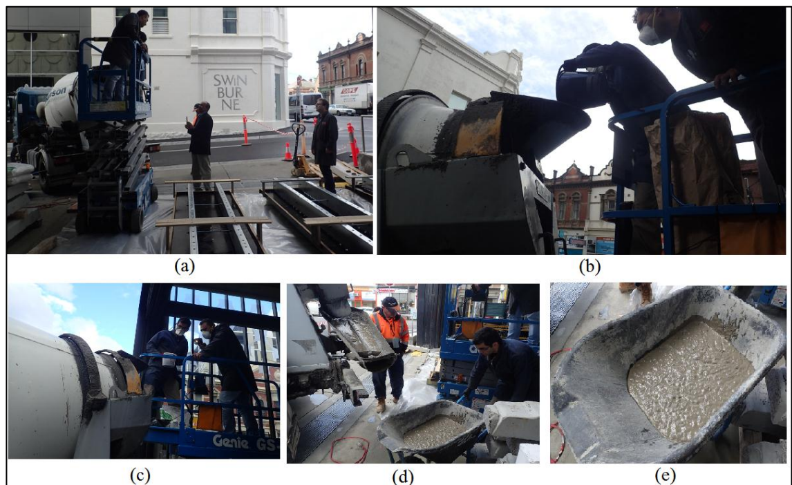
Figure 12-15: Different stages of the mixing procedure, (a): arrival of mini-truck mixer containing fly ash, slag and 80% of the needed water at the casting site, (b): addition of the PVA fibers gradually, (c): addition of the solid activator and remaining water gradually, (d) and (e): appearance of fresh composite ready for casting
