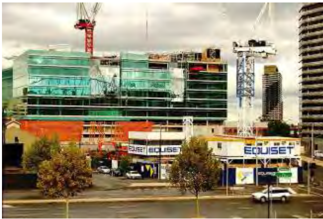
Figure 6.5: The AXA Group building
