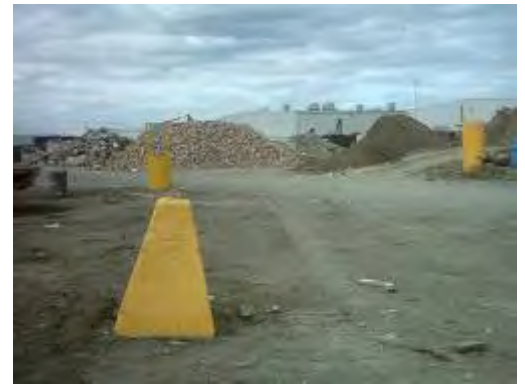
Figure A5.3: Piles of C&D waste
