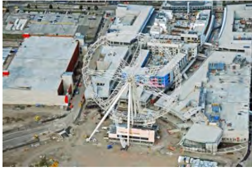
Figure 6.6: An aerial view of the Waterfront city showing the observation wheel in the foreground
