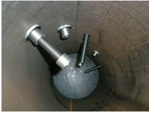
Figure 3 Blind bolts in the CHS
