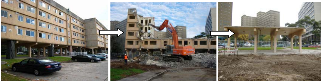
Figure 5. Demolition process of the buildings.
