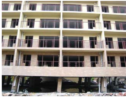
Figure 2. Soft first storey of 6-storeys building in Dujiangyan with drift of about 7.5%
